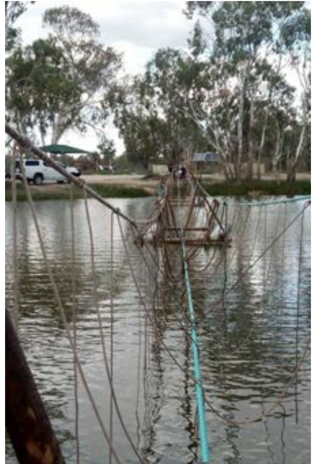
Bridge constructed by participants
